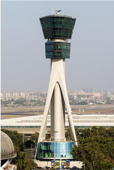
Figure 45 Air control center
